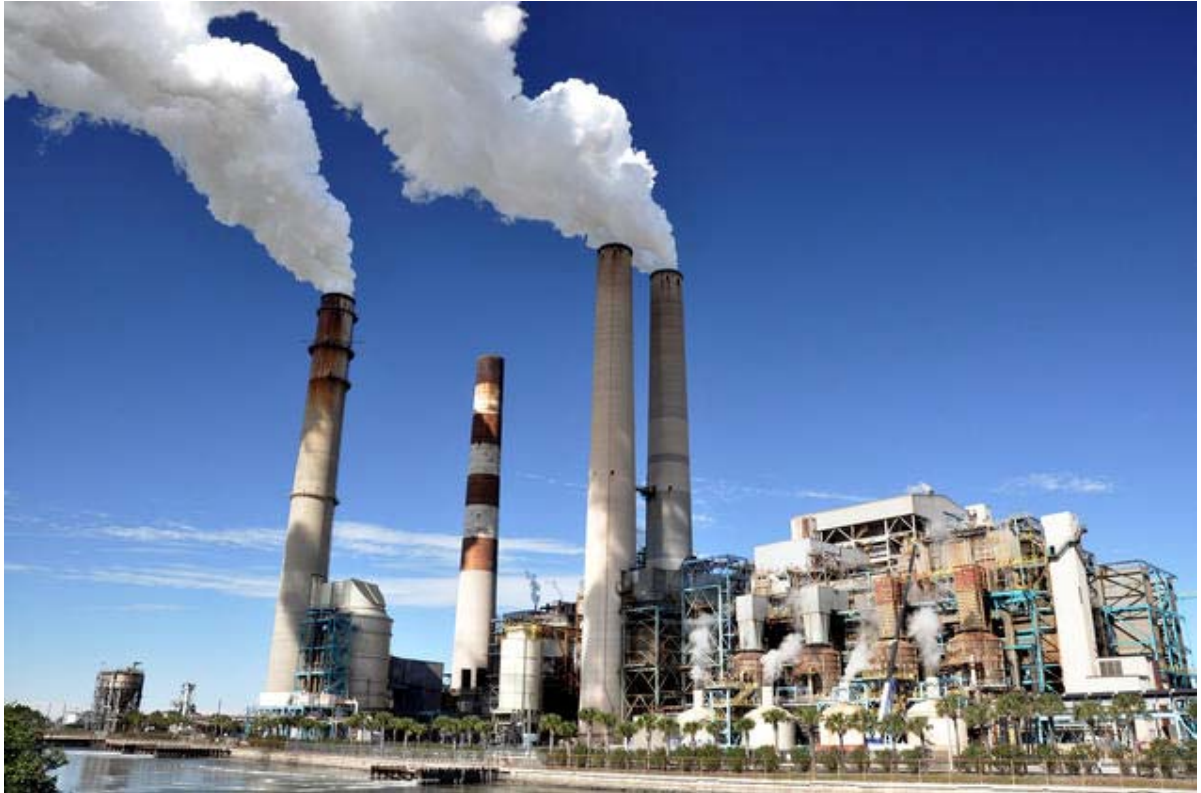
Big Bend Power Station, a coal-fired power plant in Tampa, Florida
